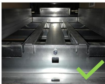
Support profiles correctly installed
